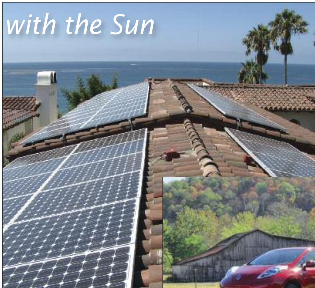
Candelaria Solar Electric recently installed this 12 kW solar power system in San Clemente.
